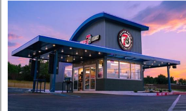
7BREW WHITE HOUSE TN Indoor & Outdoor Electrical Installations Parking Lot and Pole Lighting Systems Utility Primary and Secondary Electrical Infrastructure
