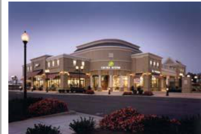
KIMCO FACILITY MANAGEMENT MT JULIET TN Office electrical work Main Panel Relocation
