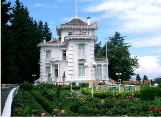
ATATÜRK MANSION LV panel building and installation works.
