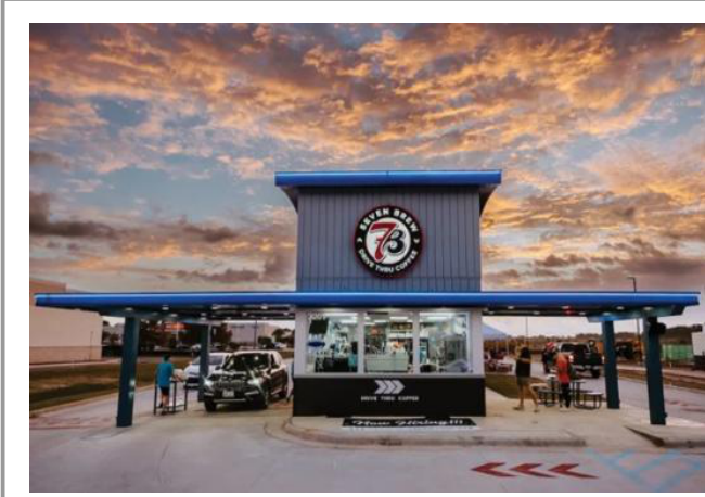
7BREW LA VERGNE TN Indoor & Outdoor Electrical Installations Parking Lot and Pole Lighting Systems Utility Primary and Secondary Electrical Infrastructure
